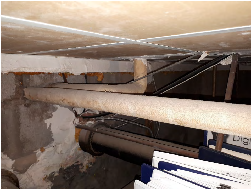
Photo 7 – Pipe insulation in the basement of the club house observed to be fiberglass.
