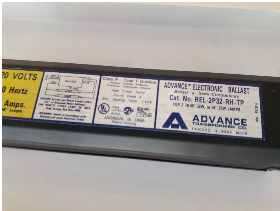
Photo 4 – Light ballast inspected from 2 nd floor common room. No PCB's identified.
