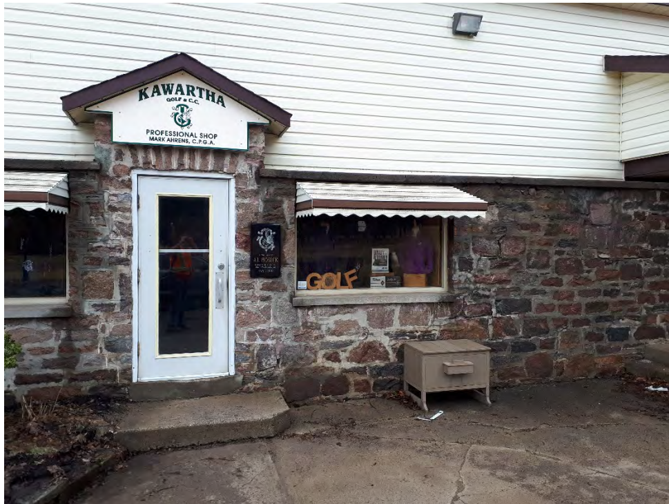
Photo 9 – View of Pro Shop building.
